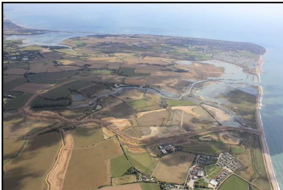
Figure 2.2: Medmerry Realignment shortly after breaching (September 2013) also showing Bunn Leisure island breakwaters near to the breach
