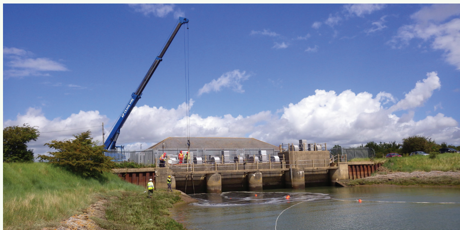
View of Hobhole Pumping Station during eel passage research in 2015 (Martin Redding)
