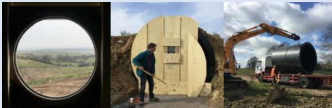
The Reveal being installed. Photo credit: Jo Sampson
