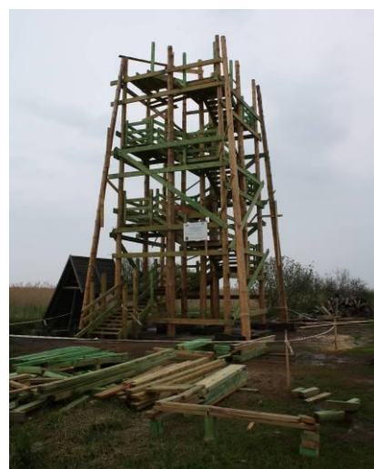
Plate 1: Observation Tower under construction, Kluki, Slowinski National Park
